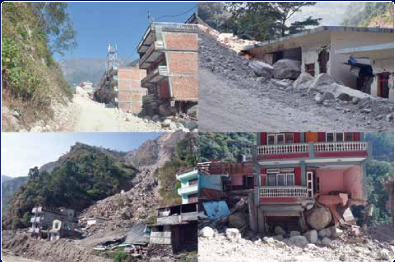
Figure 11: New settlements along the Kodari Highway were severely damaged by earthquake-induced landslides
